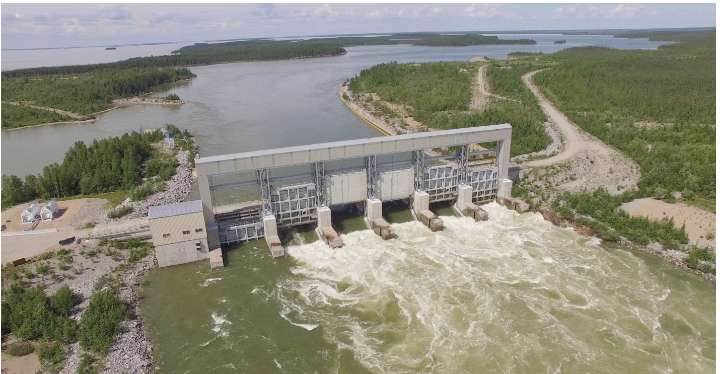
The Missi Falls Control Structure during a sudden and extreme release of water down the Lower Churchill, June 2020. Photo courtesy of Michael Tyas / Wa Ni Ska Tan
